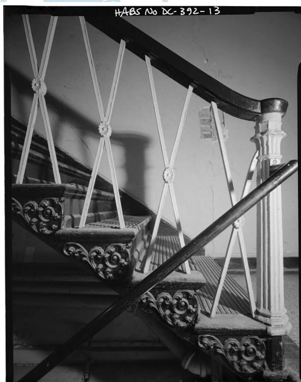
INTERIOR DETAIL, CAST-IRON STAIRWAY - Winder Building, Seventeenth & F Streets, Northwest, Washington, District of Columbia, DC
