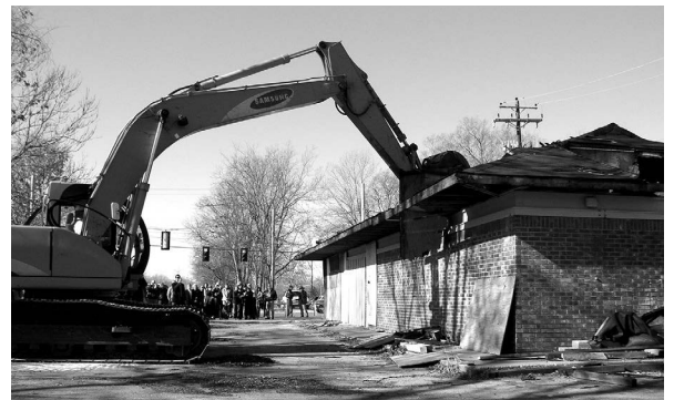
Demolition of the Pizza Hut in 2005. ©The Battle of Franklin Trust
