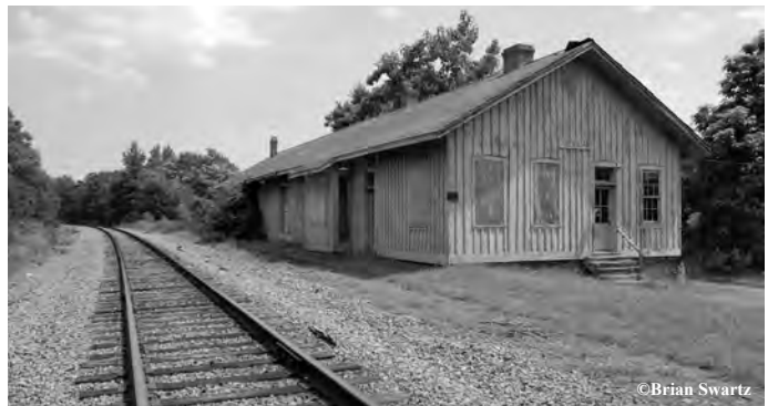
Structure west of the site of the Trevilian Station depot.
