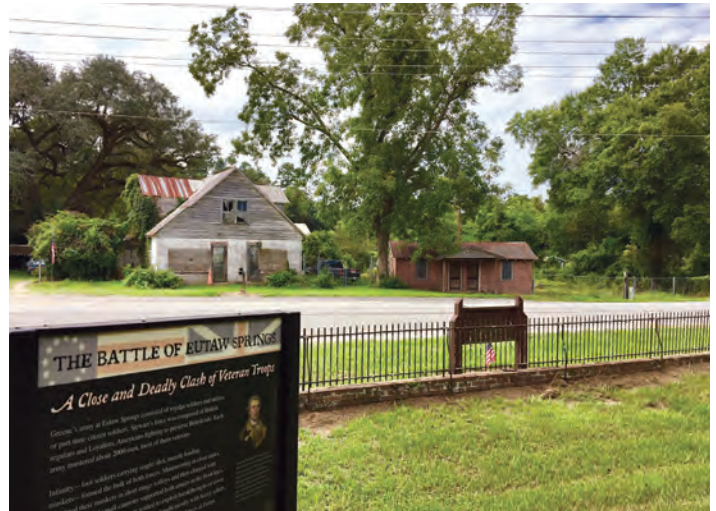
Eutaw Springs Battleground Park overlooks a deteriorating house that has become an eyesore near this hallowed battleground.
