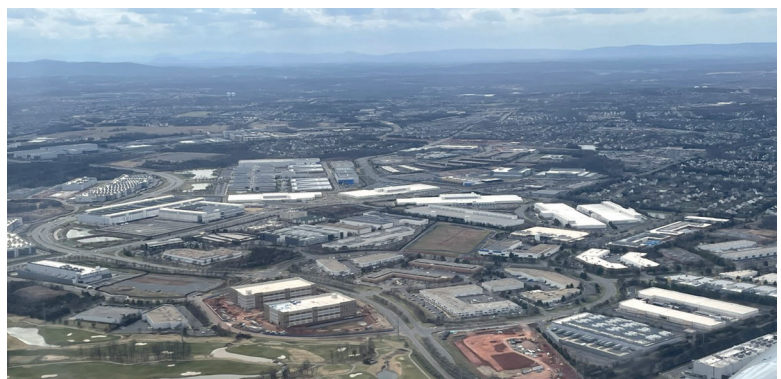
Aerial view of data centers in Loudon County — Northern Virginia.
